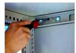
Inside fixation by nuts to avoid accident
